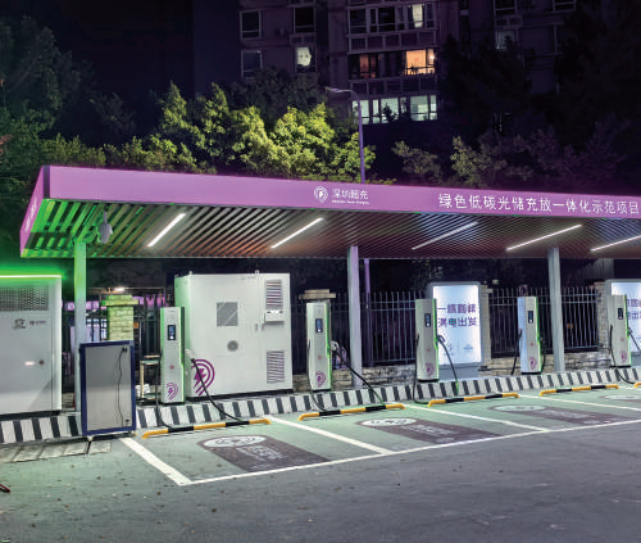
• China 100kW/215kWh DH200F Peak-to-valley arbitrage + Peak-shaving
