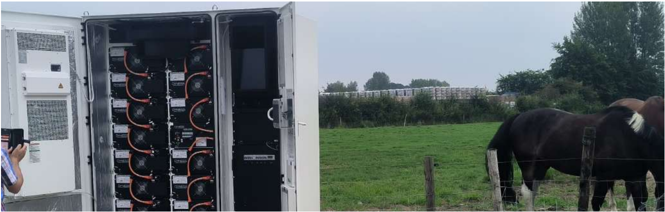
• The Netherlands 100kW/215kWh DH200F PV consumption (self-use)
