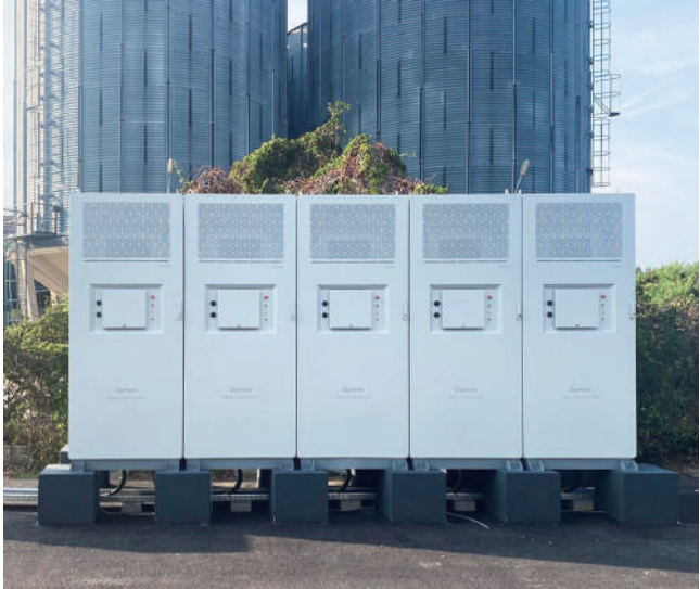
• Hungary 500kW/1160kWh DH200Y Self-generation and self-use+PV consumption
